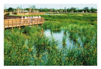
Constructed wetlands provide a natural process to remove pollutants from urban runoff
