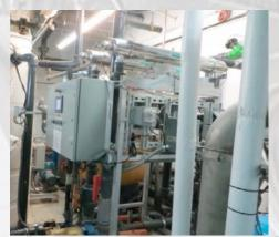
Disinfection apparatus and System Controller
